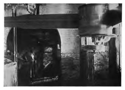
Unprotected Transmission Belt Less than Six Feet from the Ground.
